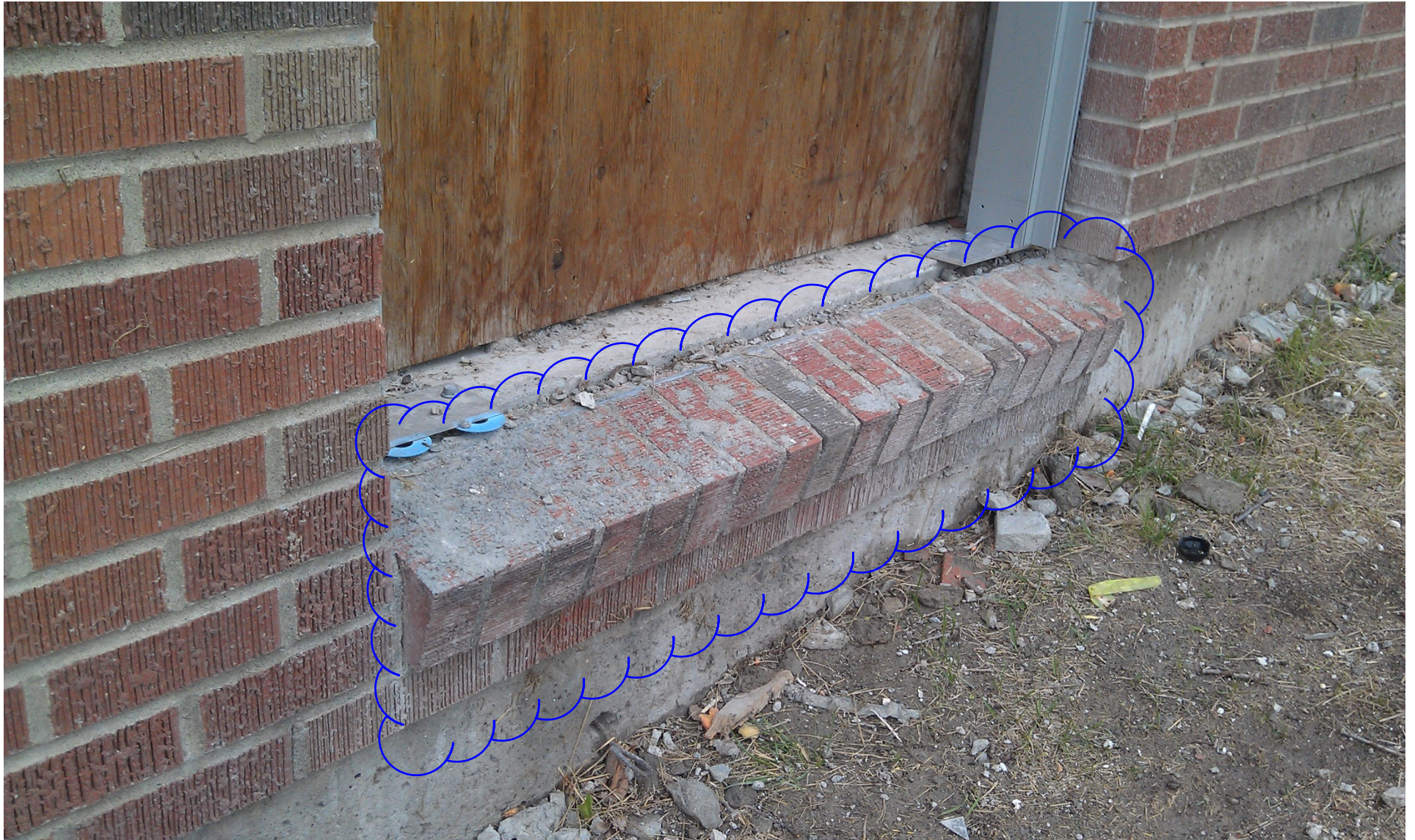
REMOVE BRICK SILL AND BOTTOM COURSE FROM CONCRETE FOUNDATION
